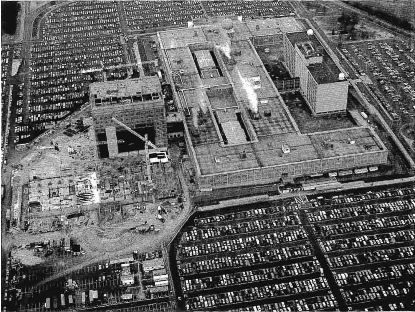
(U) Construction of Ops 2A
